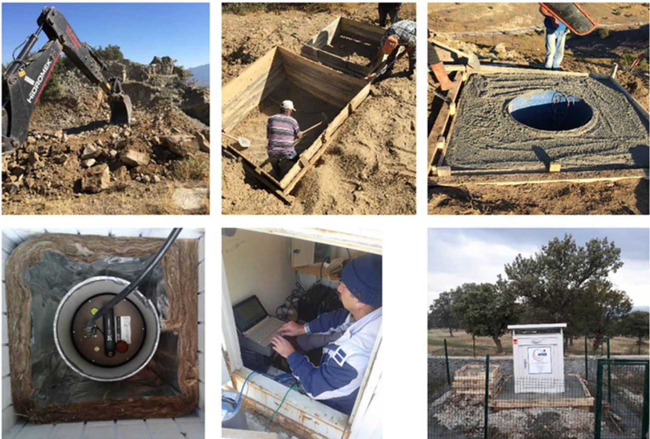
Figure 5.9: Station installation in the field (seismometer).
