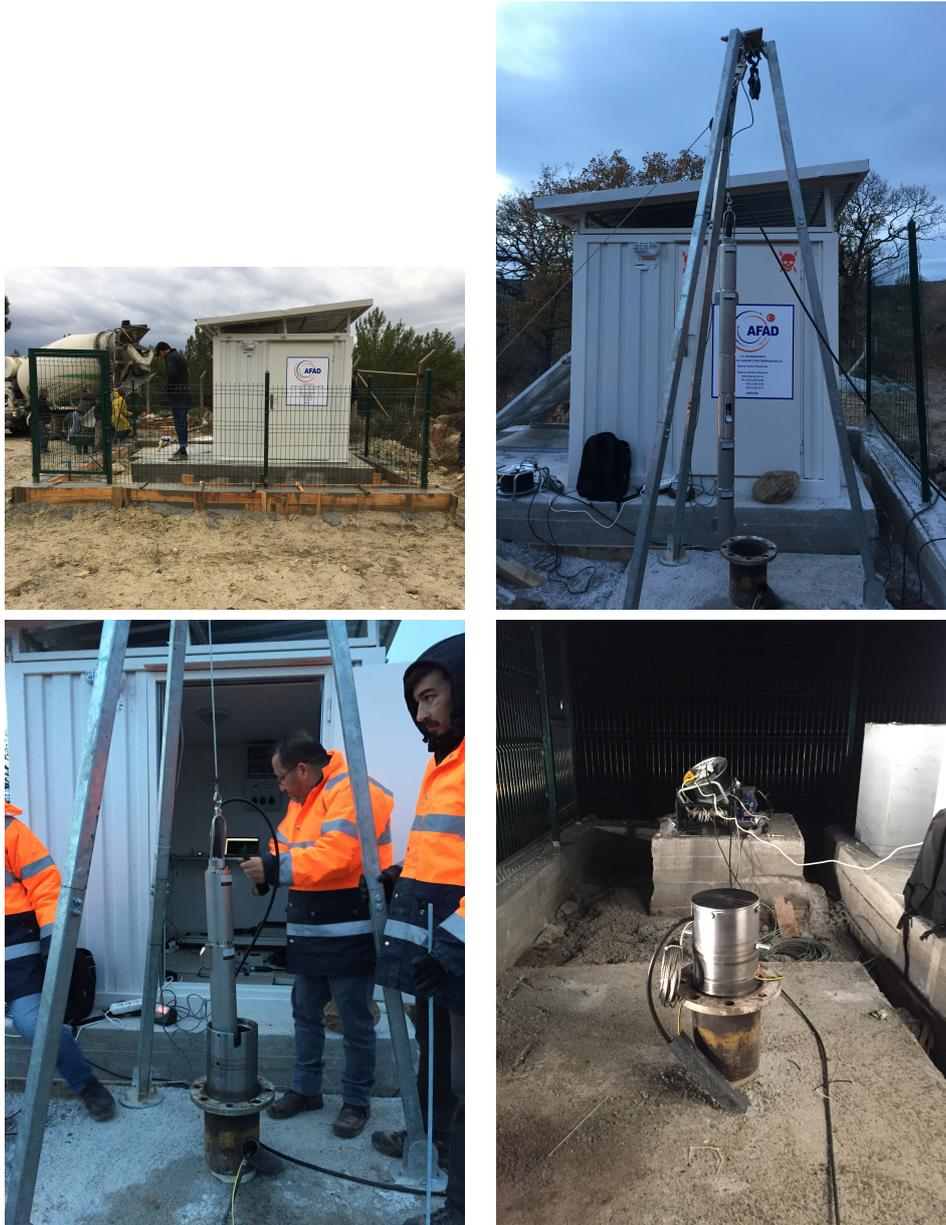
*Figure 5.14: Borehole station installation.*
