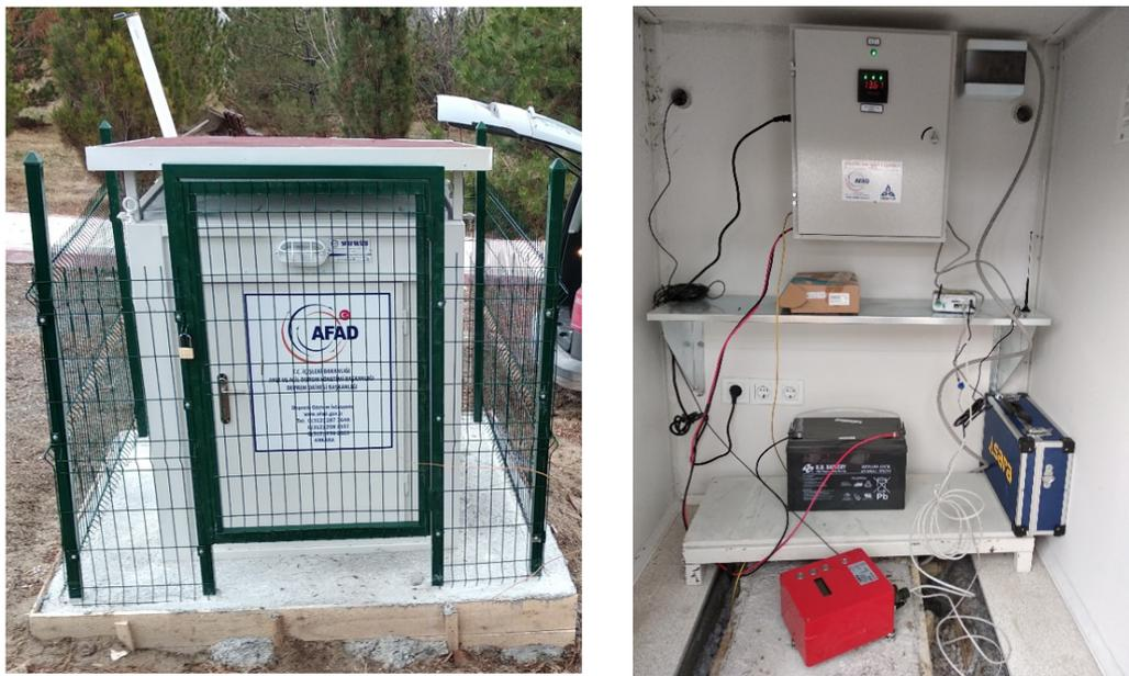
Figure 5.12: Example of a strong motion station.
