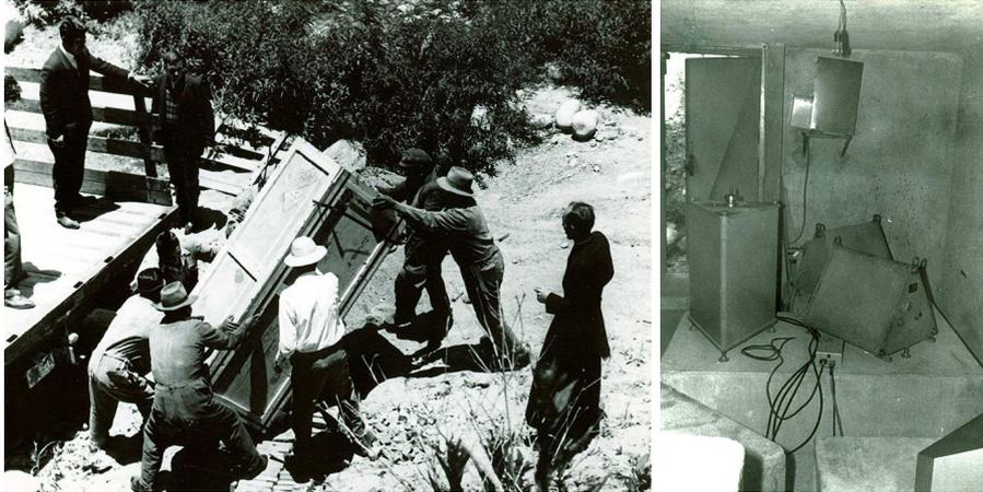
**Figure 5.3:** Left: LPB installation at Seguencoma, La Paz - Department, Right: Benioff short period seismometer at Seguencoma. (Minaya et al., 2013).
